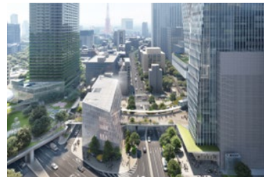
20m-wide pedestrian deck connecting across Toranomon
