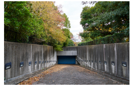
UNDERGROUND PARKING LOT (WITHIN AOMI MINAMI PORT PARK) Started to use in April 1997, this parking facility with an area of 7,603.75 square meters accommodates 216 vehicles. This underground space, currently not in use, will be opened for a limited period as an exhibition venue.
